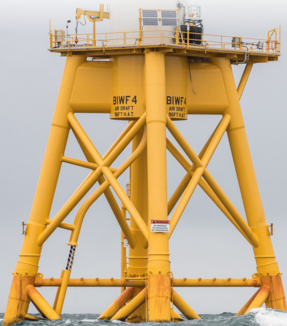
Photo by Dennis Schroeder, NREL 40465
