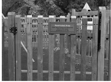
Photograph 5. Childproof lock on the gate of the Liberty Swing enclosure
